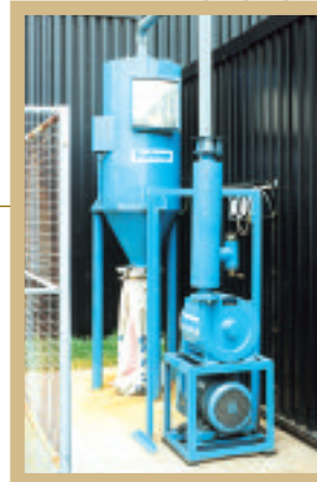
Typical vacuum cleaning system with 6X7 Turbo exhauster driven by 11Kw motor, providing the suction power.
